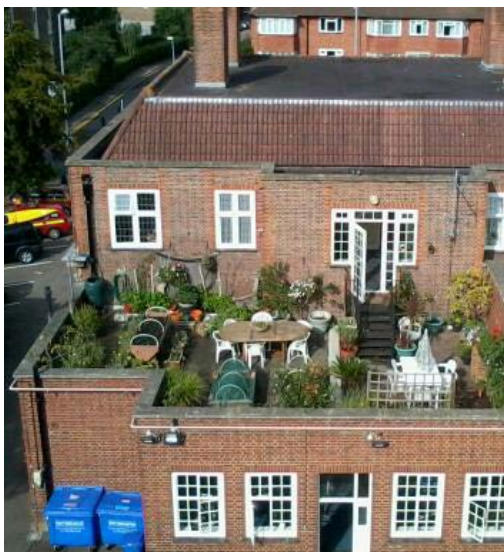
Surbiton Fire Station roof allotment
